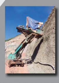
Supplying machines and equipment for the execution of rock bolts anchors and tendons in the berms and walls of the section of left side RAGHOON dam in TAJIKESTAN.
