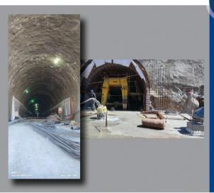
Design, supply of equipment, materials and implementation of the project of tunnel and channel for the transfer of lang materials from SARCHESHME copper factory and DAREHZAR copper factory (tunnel slop: 23%) in IRAN to the location of the flotation plant (Engineering Procurement Construction)
